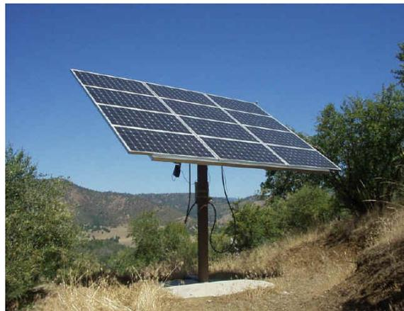
Figure 1. Two Axis Solar Tracker
